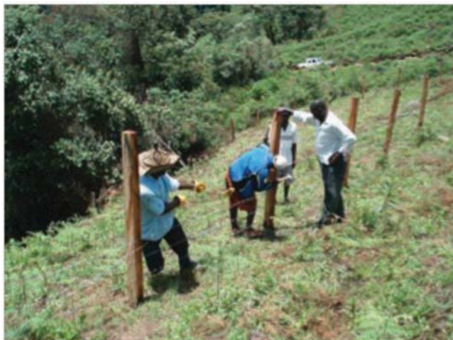
FIGURE 5.7: Tensioning Barbed Wire and Nailing a Dead Fence
