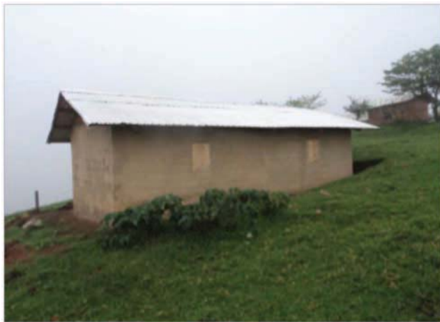
FIGURE 10.4: Another View of Secondary Building
