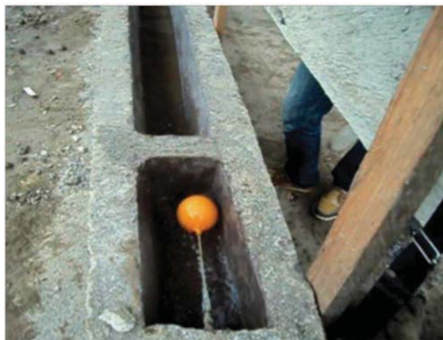
FIGURE 10.9: Drinking Trough and Water Control System
