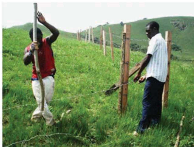
FIGURE 5.8: Constructing a Fence Gate
